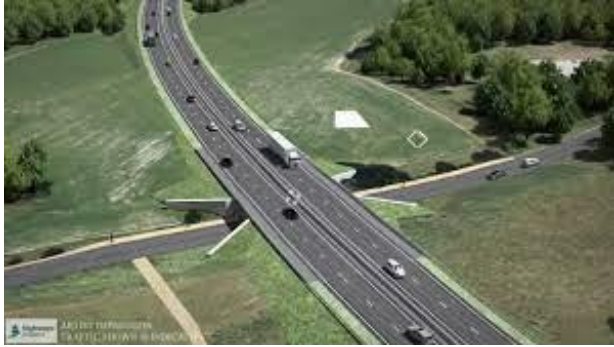
A27 Arundel Bypass
