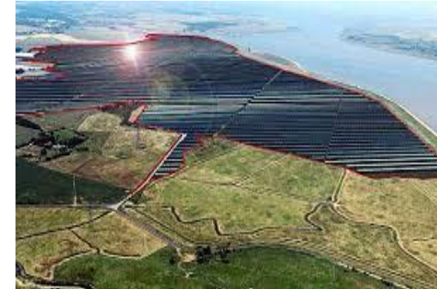
Cleve Hill Solar Park
